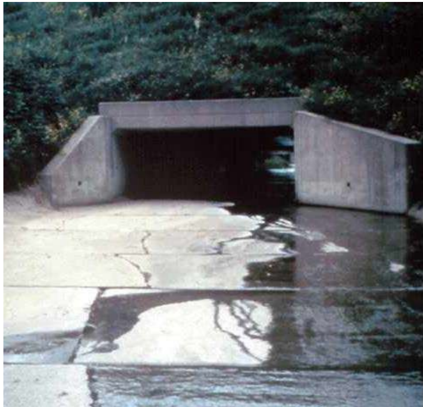
Figure 13.1.15 Formed Concrete Channel Lining
