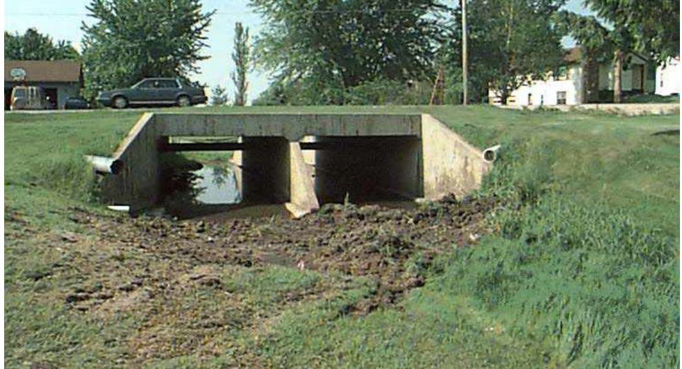
Figure 14.2.8 Concrete Frame Culvert
