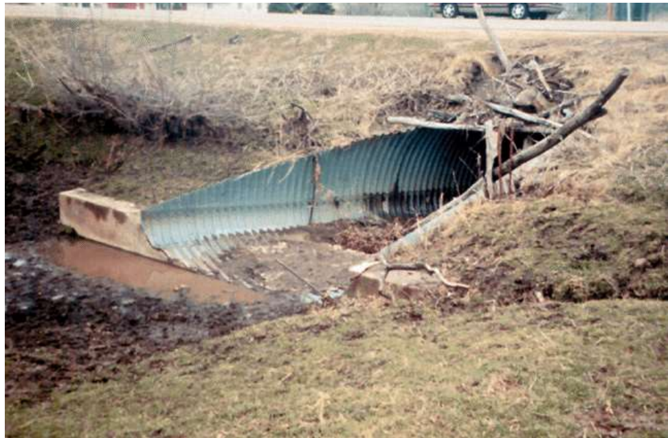
Figure 14.1.19 Culvert Mitered End
