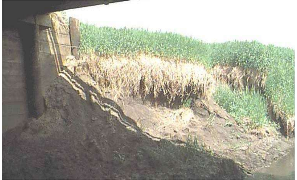
Figure 13.2.20 Undermined Streambank
