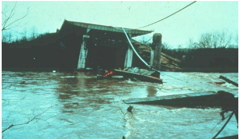
Figure 13.3.1 Schoharie Creek Bridge Failure
