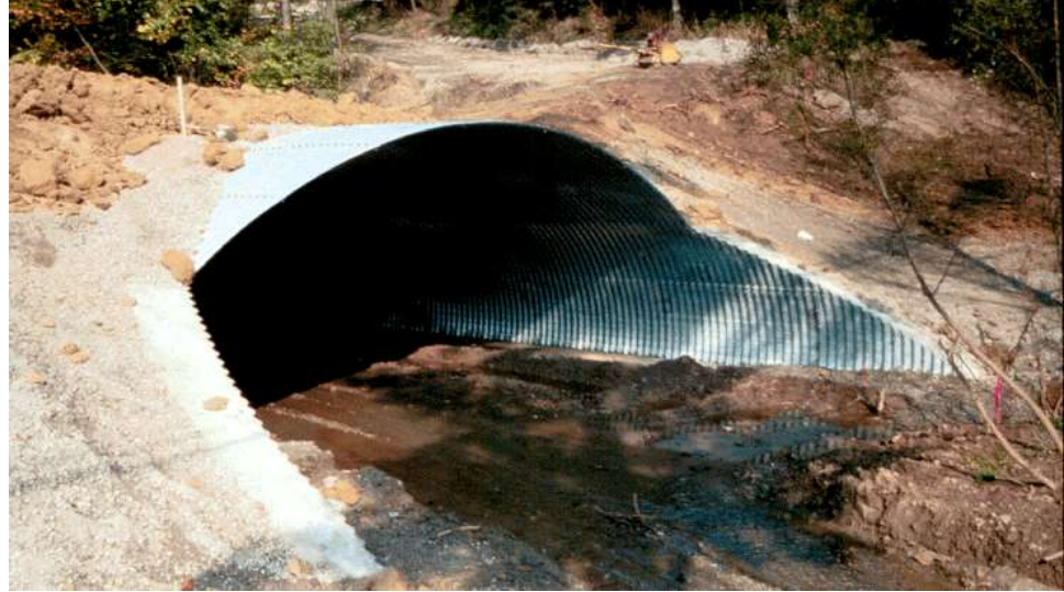
Figure 14.1.8 Pipe Arch Culvert
