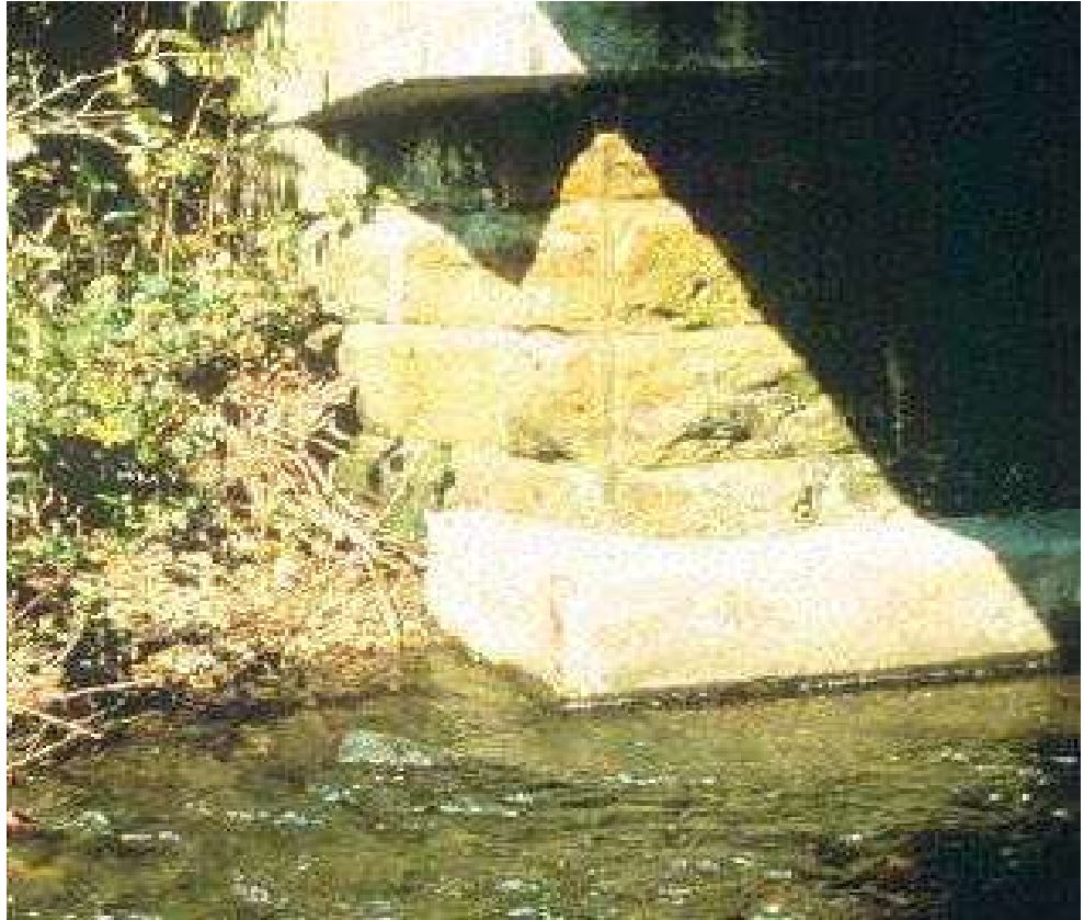
Figure 13.1.16 Concrete Footing Apron on a Masonry Abutment
