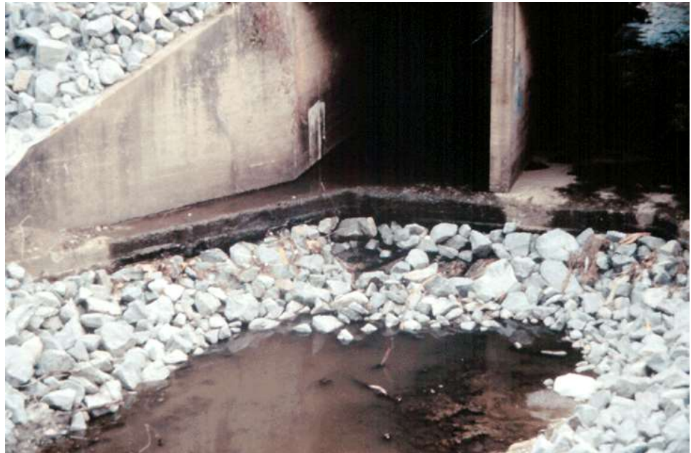
Figure 13.2.40 Failed Riprap
