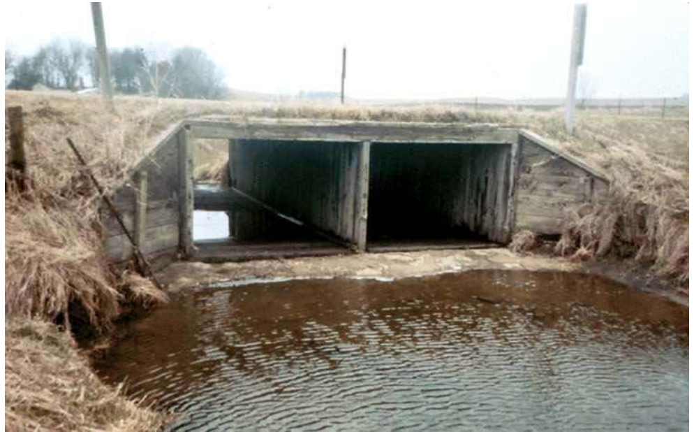
Figure 14.2.10 Timber Box Culvert
