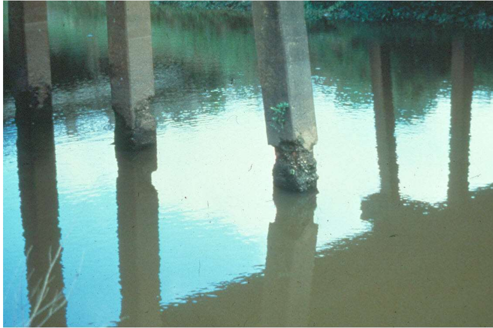
Figure 13.3.23 Concrete Deterioration
