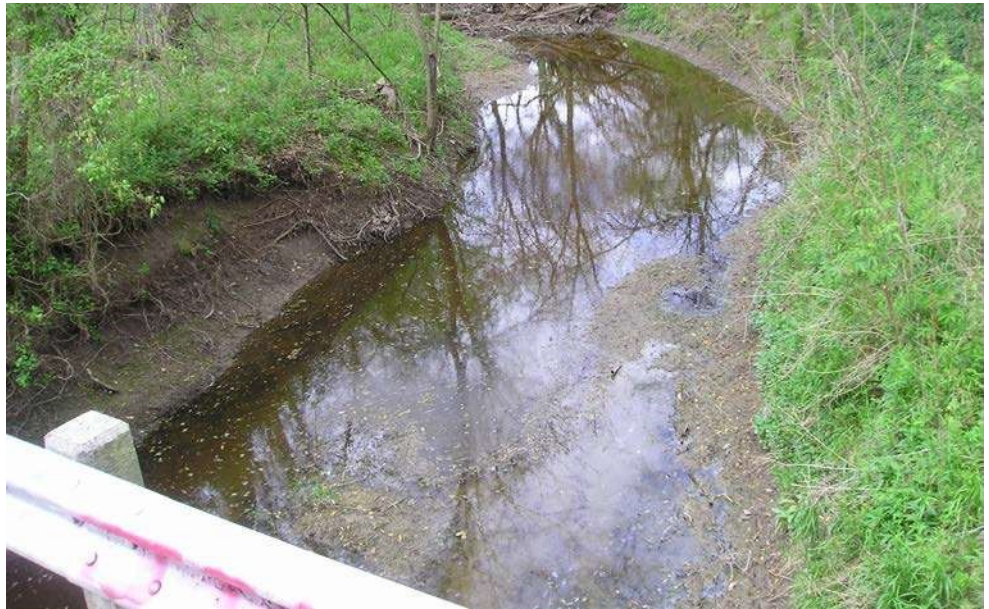
Figure 13.2.3 Streambed Degradation
