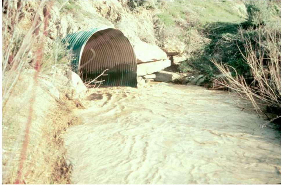
Figure 14.1.18 Culvert End Projection
