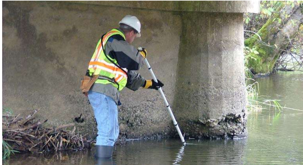
Figure 13.3.33 Inspector Performing a Wading Inspection
