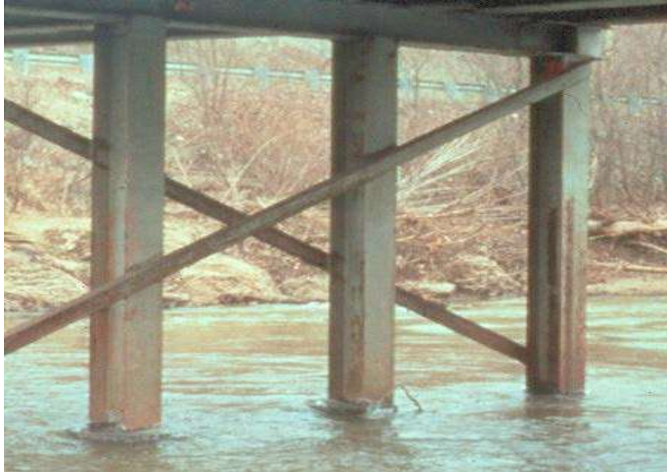
Figure 13.3.15 Steel Pile Bent
