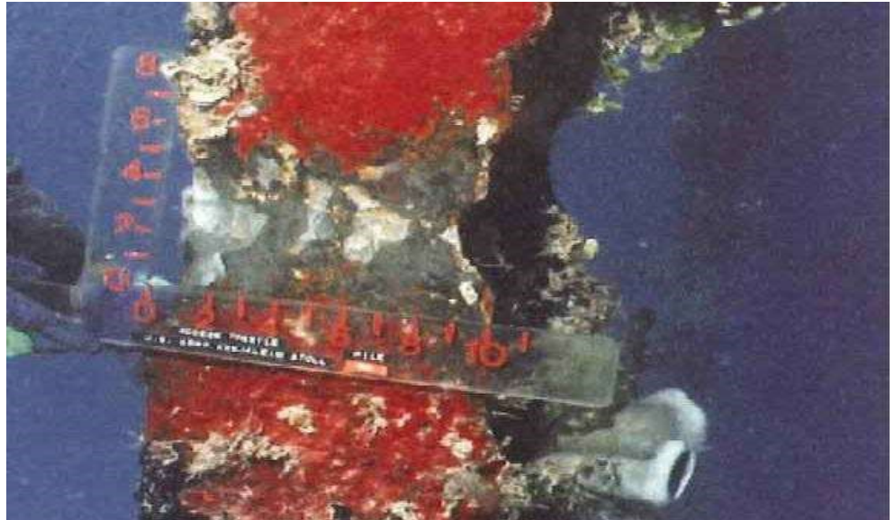
Figure 13.3.3 Level II Cleaning of a Steel Pile
