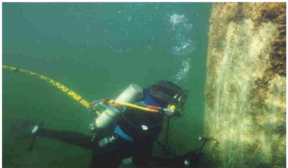
Figure 13.3.4 Diver Cleaning Pier Face For Inspection
