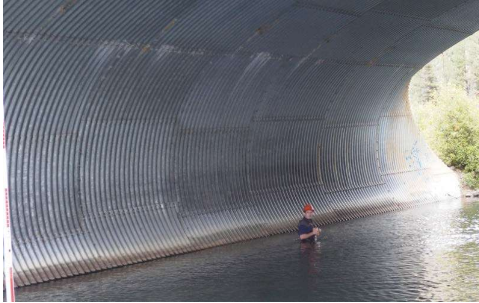
Figure 14.1.13 Large Structural Plate Pipe Arch Culvert
