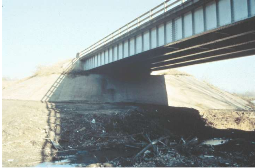
Figure 13.2.42 Approach Roadway Built in the Floodplain
