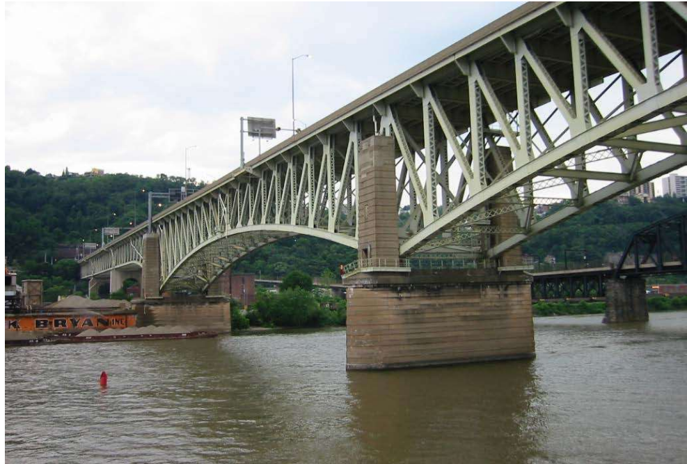
Figure 13.3.2 Liberty Bridge over Monongahela River
