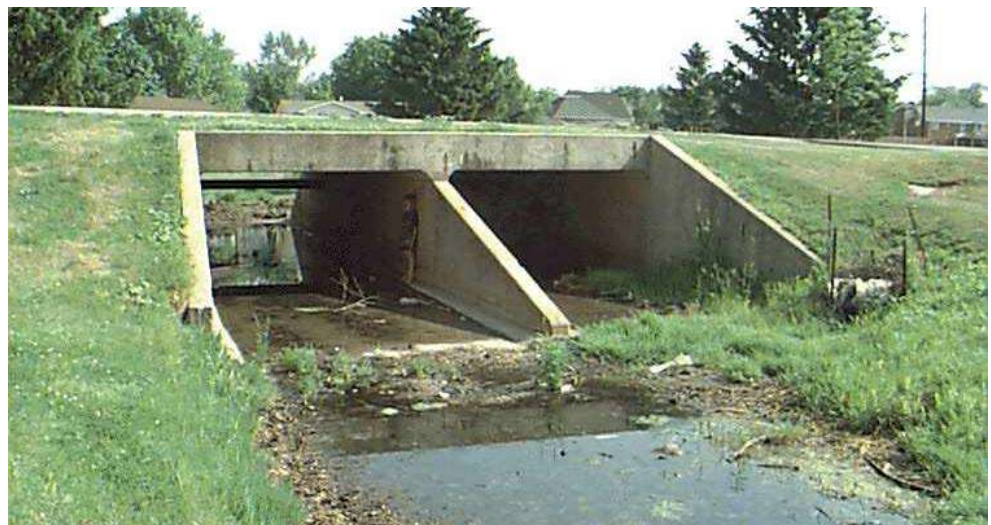
Figure 14.2.3 Multi-Cell Concrete Box Culvert
