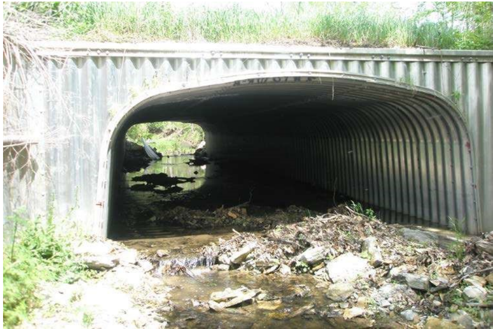
Figure 14.1.14 Large Structural Plate Box Culvert
