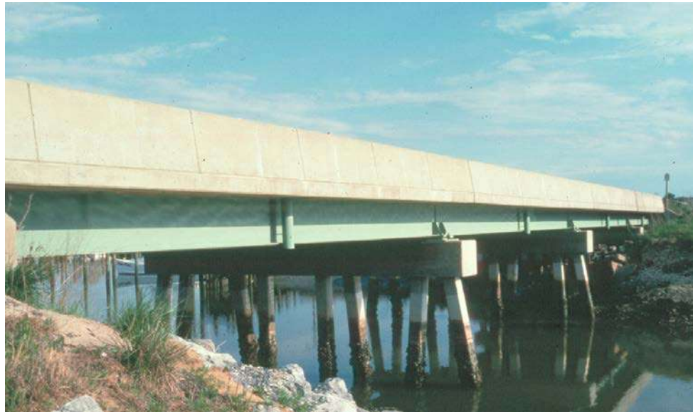
Figure 13.3.16 Concrete Pile Bent
