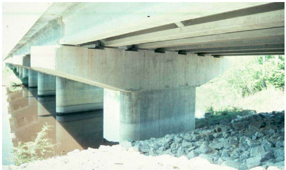
Figure 13.3.18 Cantilever or Hammerhead Pier
