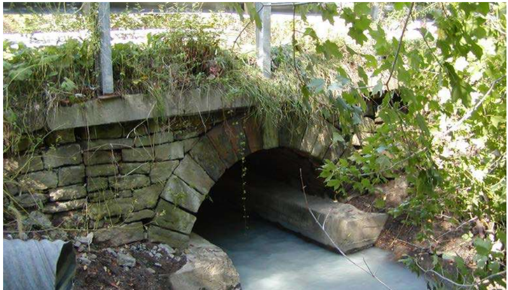
Figure 14.2.9 Stone Masonry Arch Culvert
