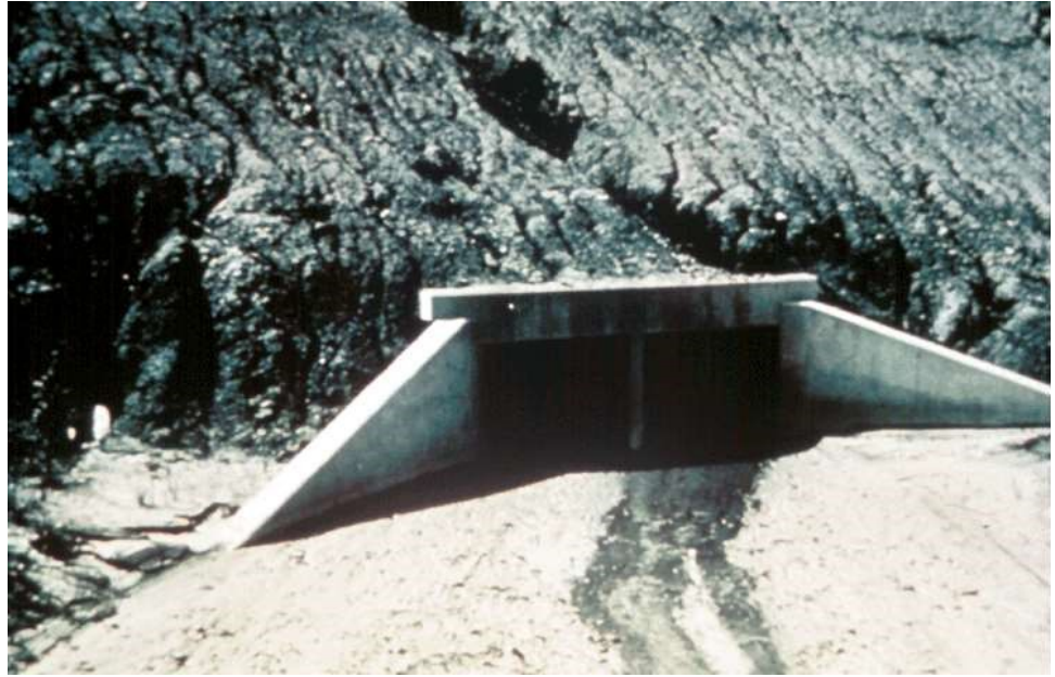
Figure 14.1.31 Slide Failure
