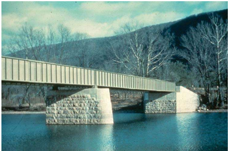
Figure 13.2.39 Multi-Span Simply Supported Bridge
