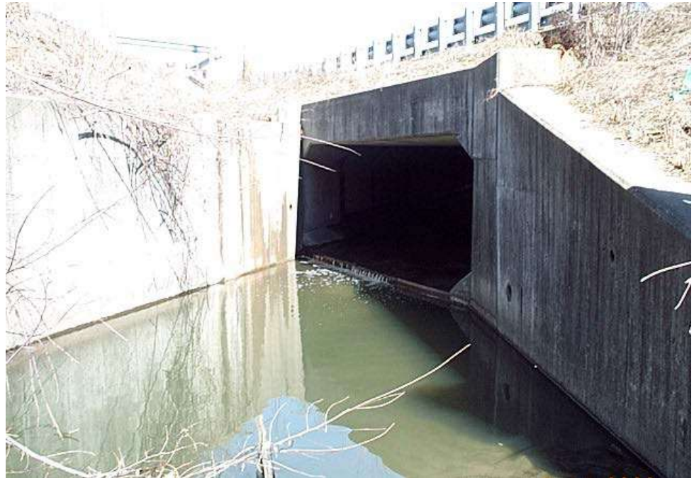
Figure 14.1.20 Culvert Skewed End
