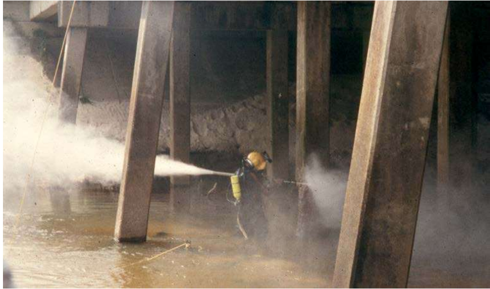
Figure 13.3.47 Cleaning with a Water Blaster
