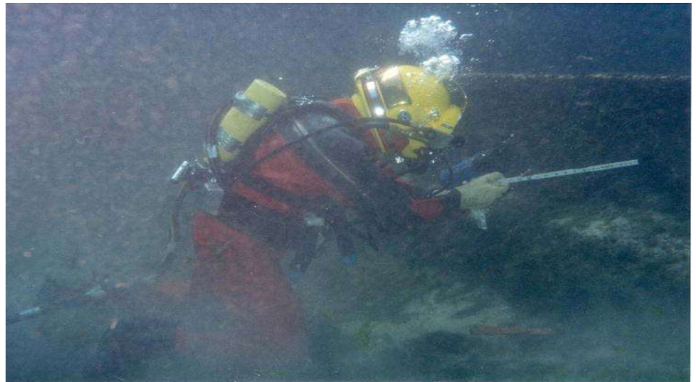
Figure 13.3.35 Surface-Supplied Diving Inspection
