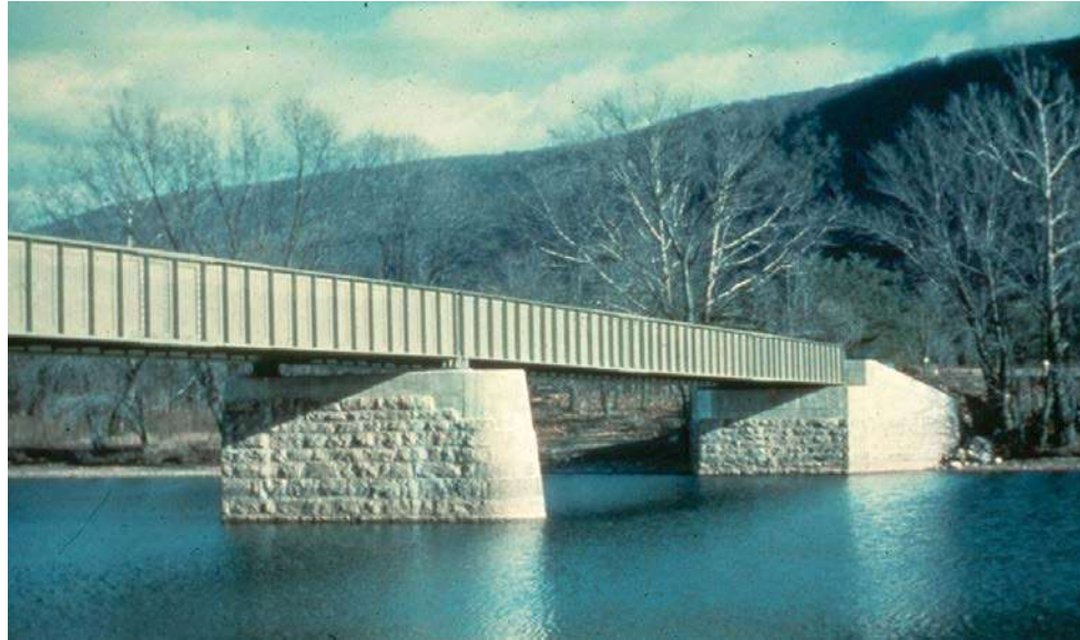
Figure 13.3.19 Solid Shaft Pier
