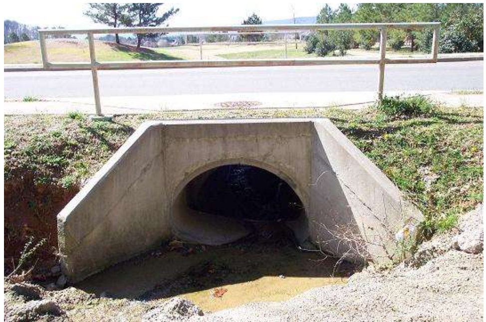
Figure 14.1.21 Culvert Headwall and Wingwalls
