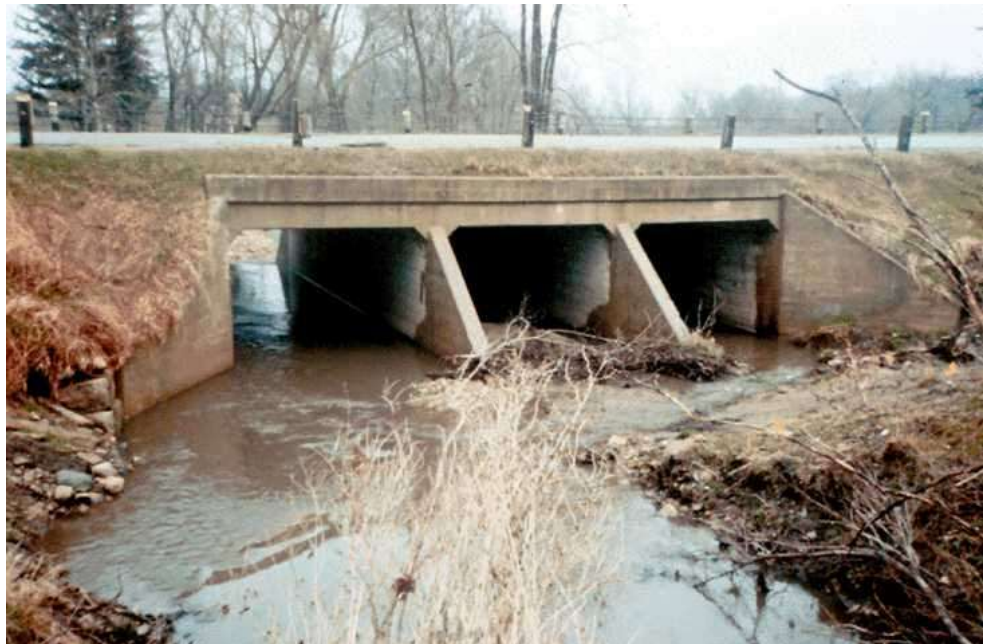
Figure 14.1.12 Frame Culvert
