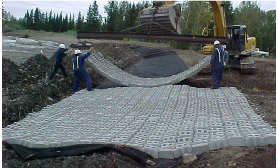
Figure 13.1.14 Concrete Revetment Mat
