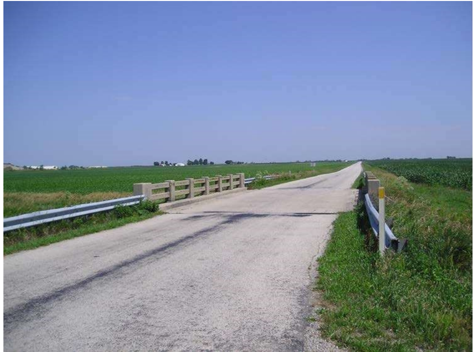
Figure 14.1.29 Approach Roadway at a Culvert Site
