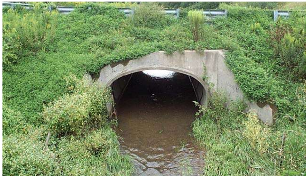
Figure 14.2.7 Concrete Arch Culvert
