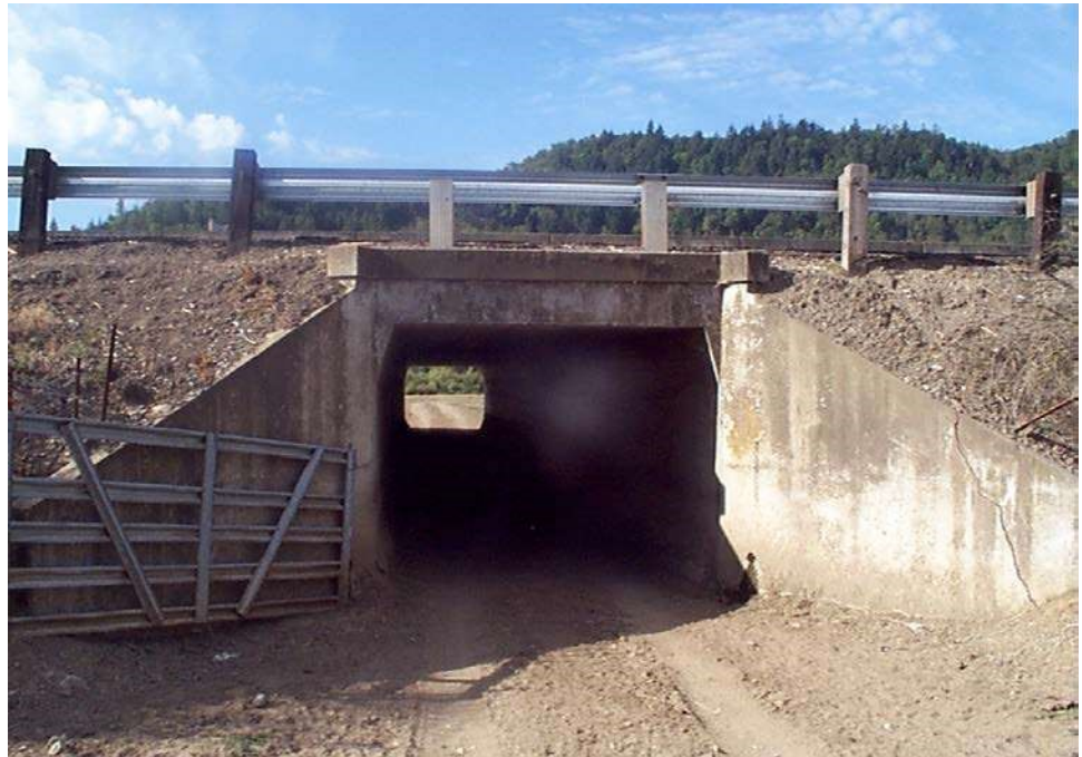
Figure 14.1.2 Box Culvert with Shallow Cover
