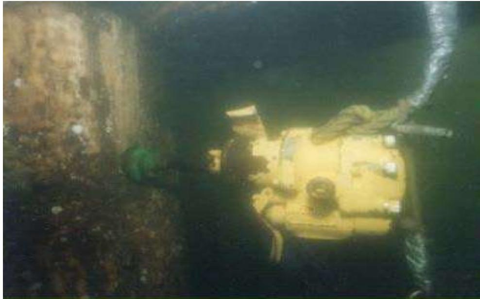
Figure 13.3.49 Concrete Coring Taking Place
