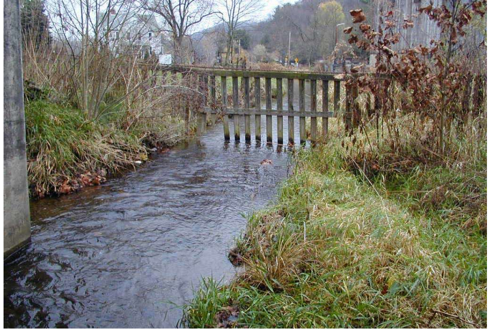
Figure 13.2.45 Fence in Stream at Bridge
