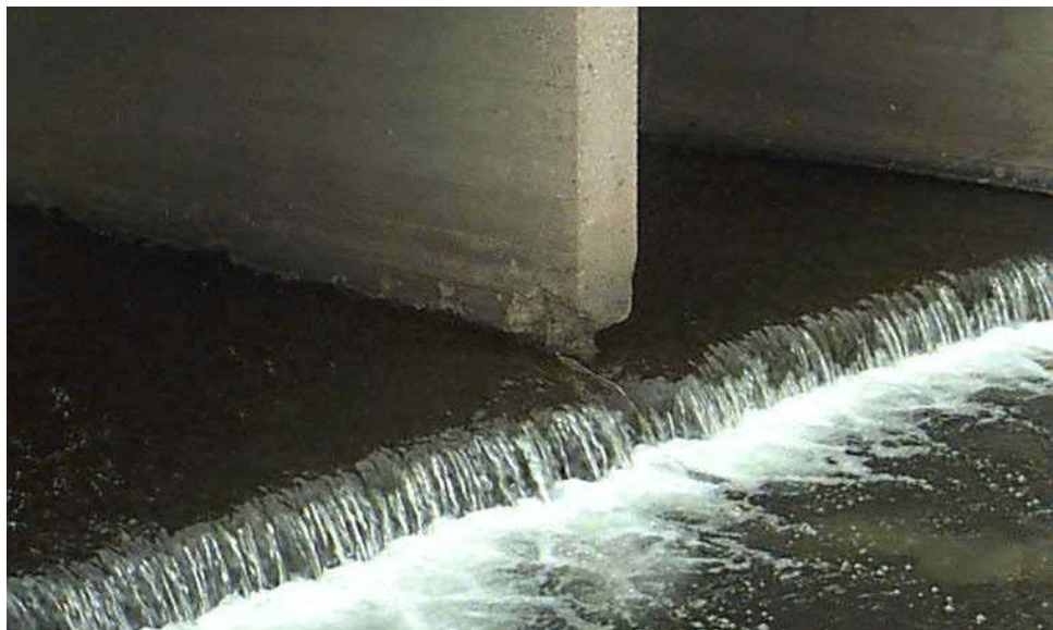
Figure 14.1.37 Energy Dissipater
