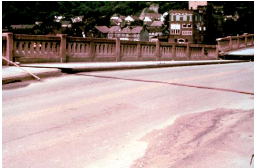
Figure 13.2.37 Superstructure Misalignment
