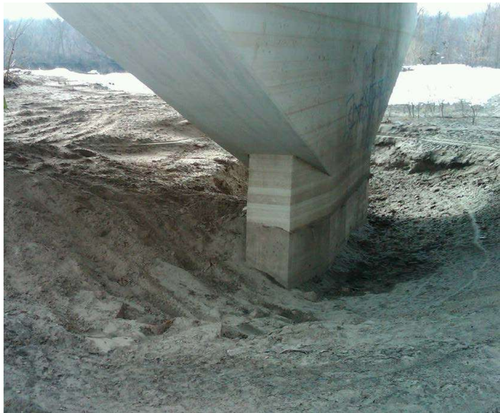
Figure 13.2.14 Local Scour at a Pier
