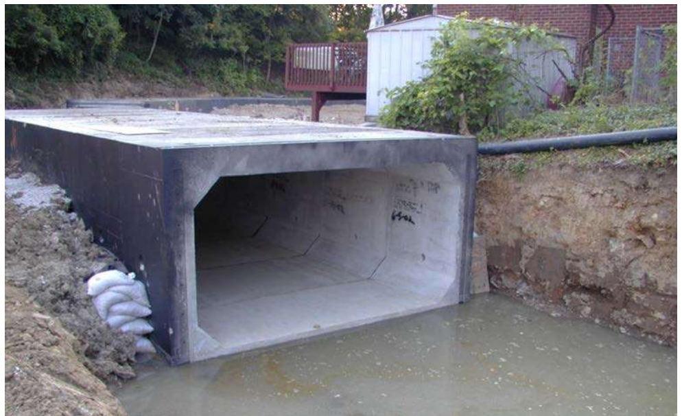
Figure 14.2.4 Precast Concrete Box Culvert
