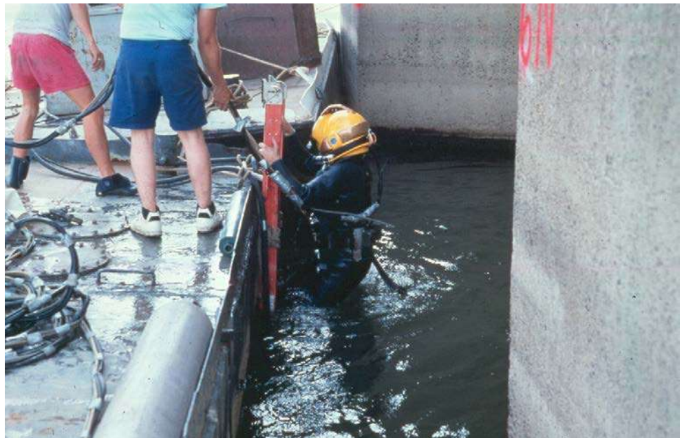
Figure 13.3.44 Access Barge and Exit Ladder
