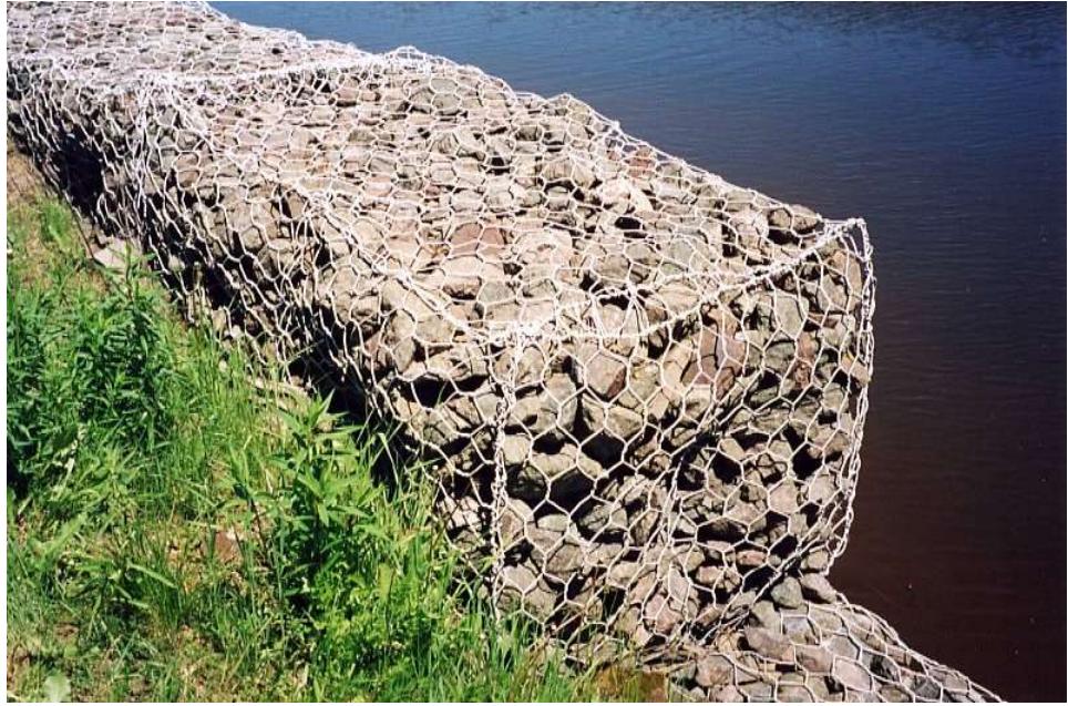
Figure 13.1.12 Gabion Basket Serving as Slope Protection
