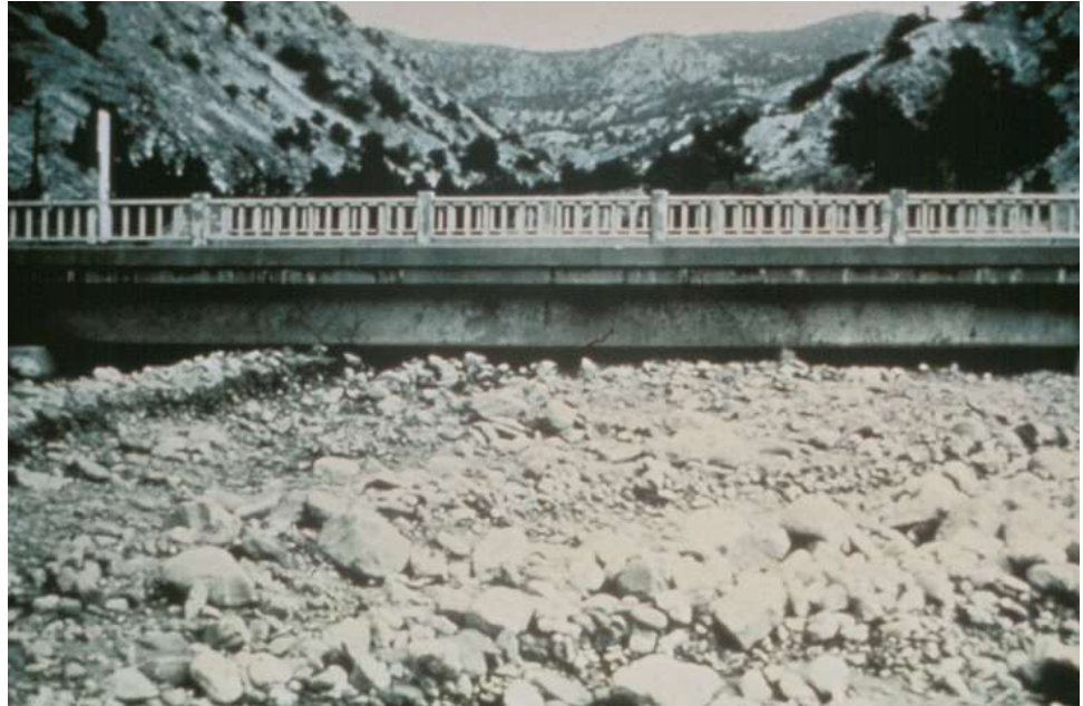
Figure 13.2.2 Streambed Aggradation
