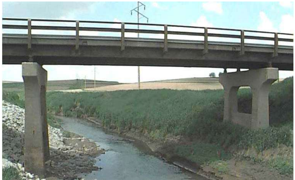
Figure 13.2.18 Streambank Damage
