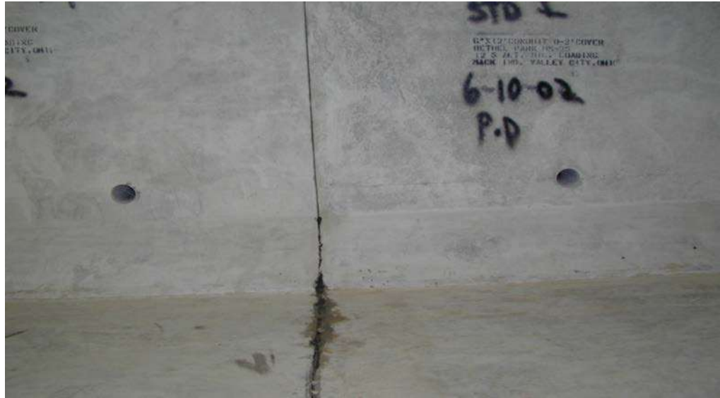
Figure 14.2.19 Precast Concrete Box Culvert Joint
