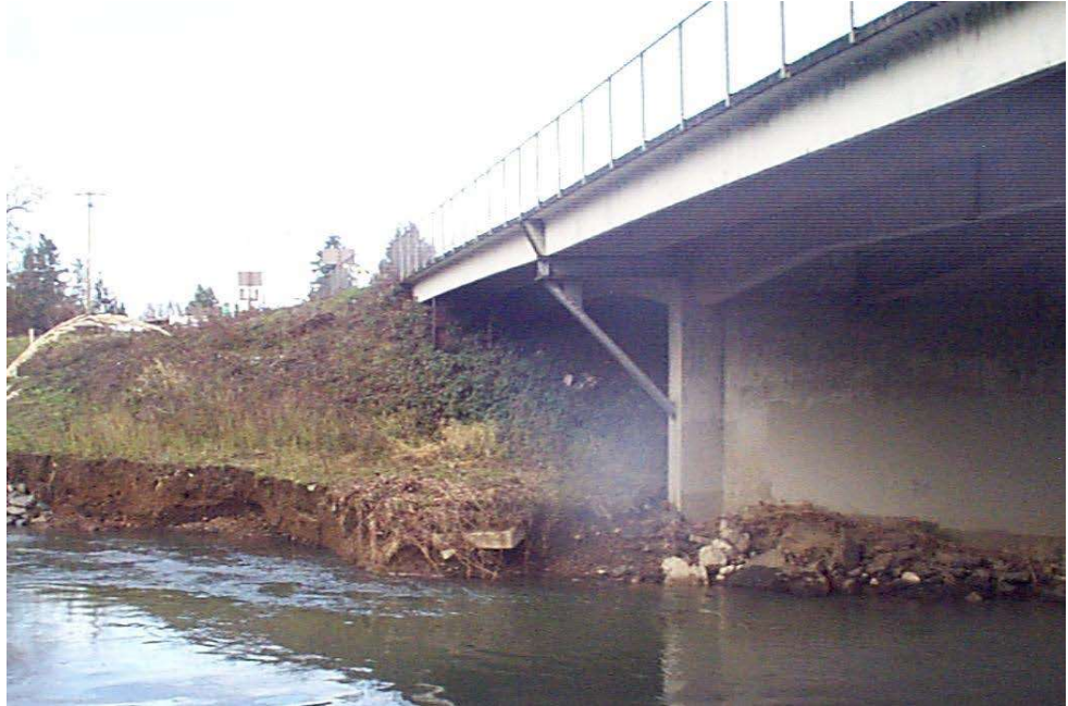
Figure 13.2.22 Channel Widening
