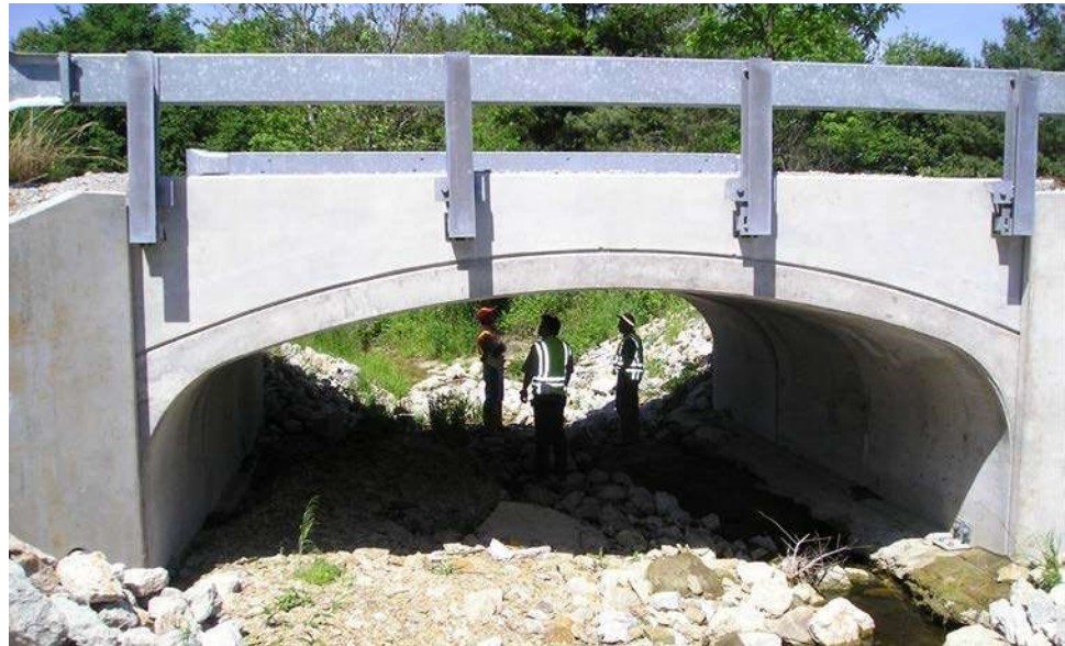
Figure 14.1.9 Arch Culvert
