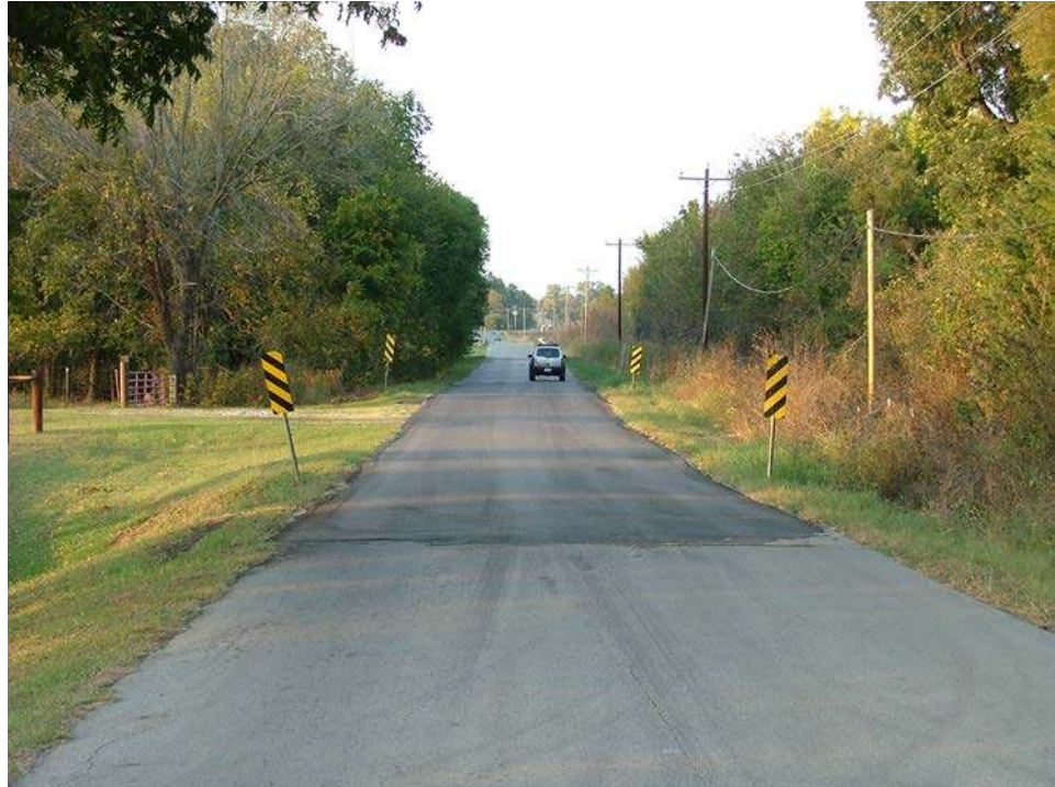
Figure 14.1.30 Repaired Roadway Over a Culvert
