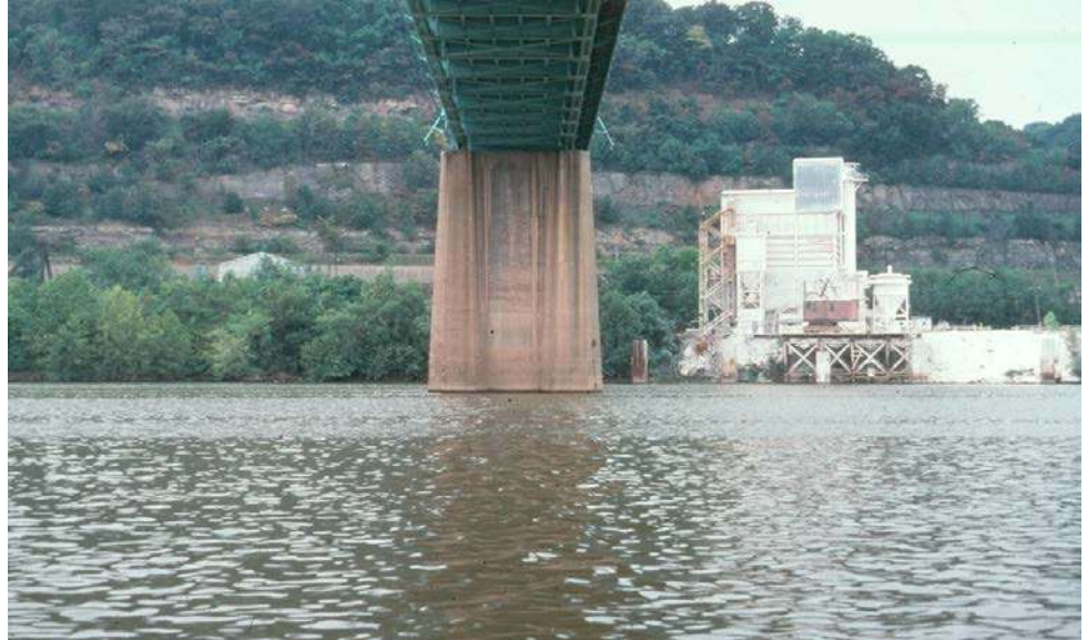
Figure 13.3.17 Column Pier with Solid Web Wall
