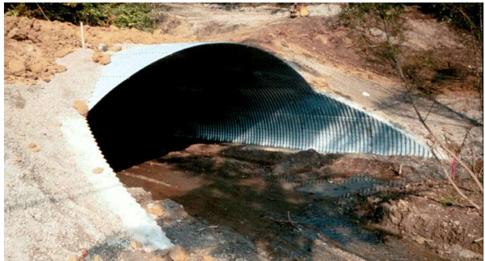
Figure 14.3.1 Pipe Arch Flexible Culvert
