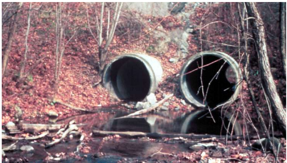
Figure 14.2.6 Twin Concrete Pipe Culvert
