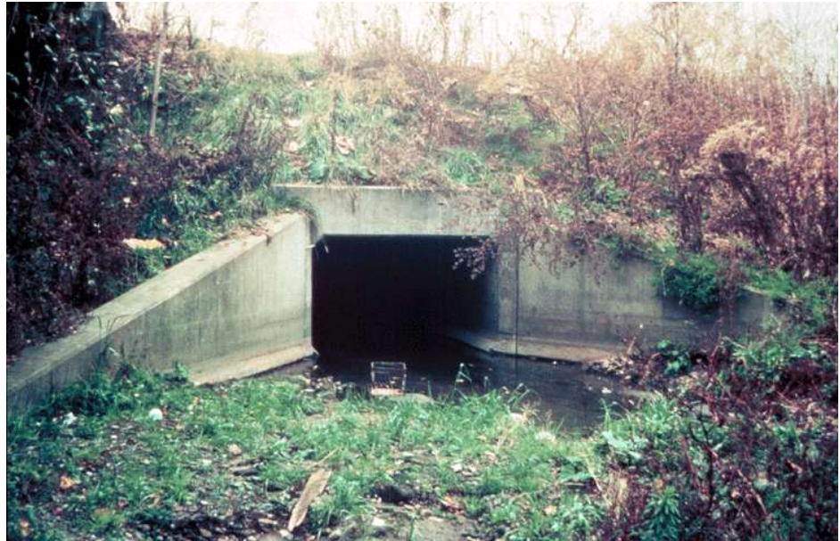
Figure 14.1.10 Concrete Box Culvert
