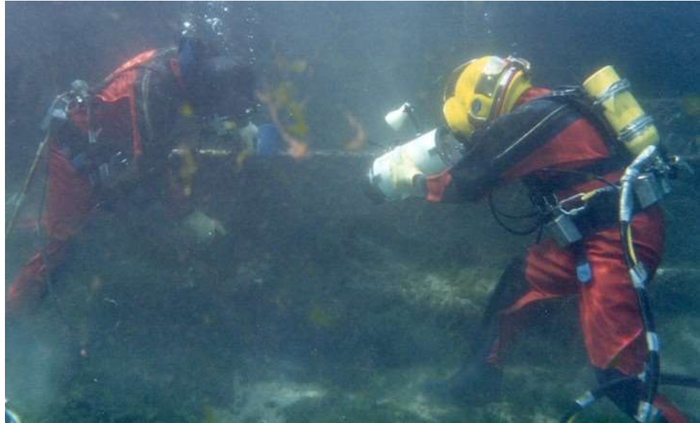
Figure 13.3.55 Underwater Video Inspection
