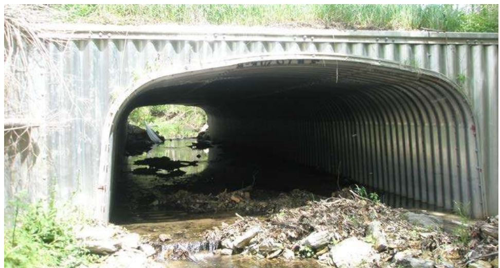
Figure 14.3.2 Flexible Box Culvert
