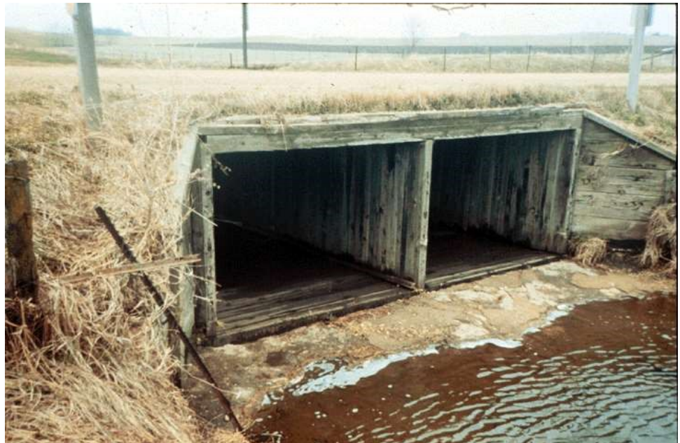
Figure 14.1.16 Timber Box Culvert
