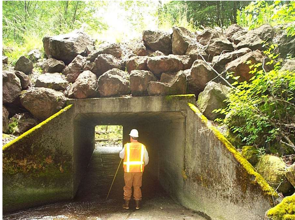
Figure 14.1.33 Potential for Tilted Wingwalls
