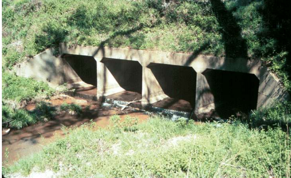
Figure 14.1.11 Multiple Cell Concrete Culvert
