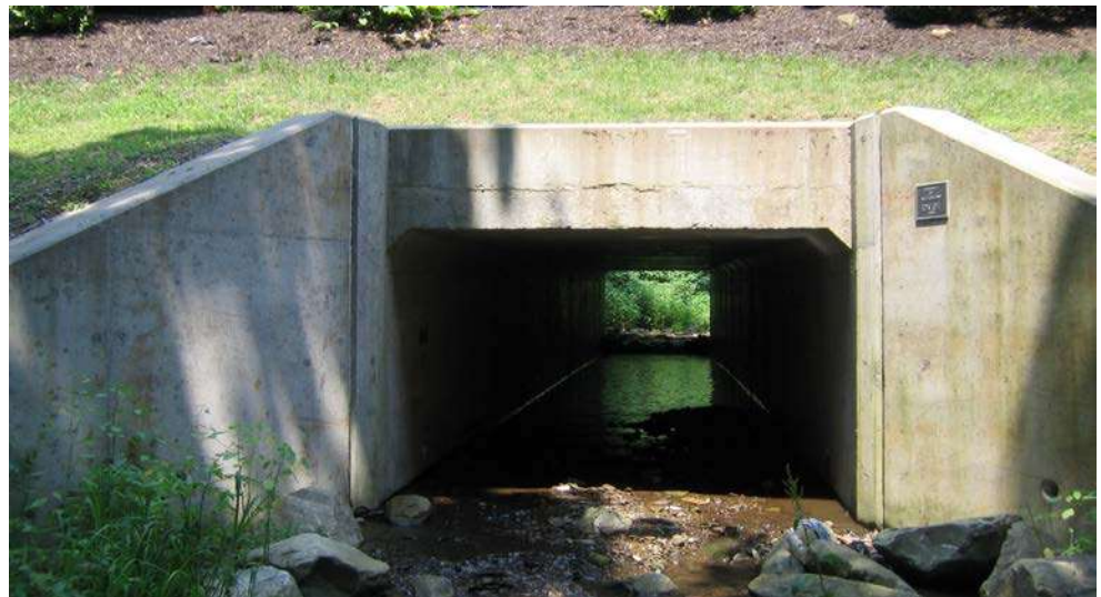
Figure 14.2.2 Concrete Box Culvert
