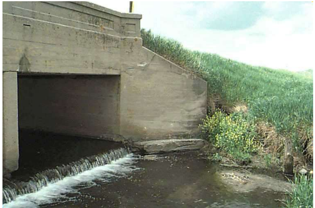
Figure 14.2.23 Cast-in-Place Concrete Headwall and Wingwall
