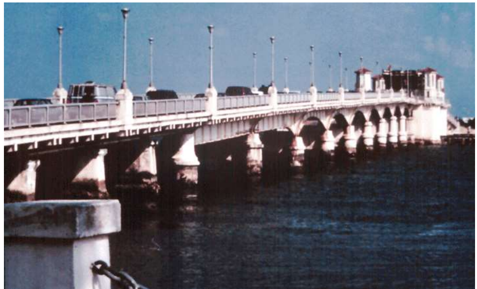
Figure 13.2.8 Large number of Piers Combine to Reduce the Hydraulic Opening
