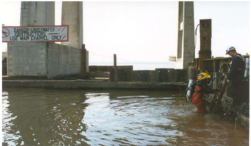
Figure 13.3.27 Diving Inside a Cofferdam
