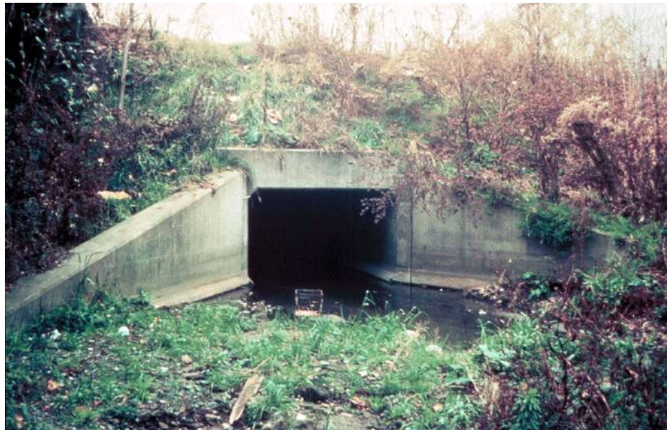
Figure 14.1.35 Culvert Headwall and Wingwall End Treatment
