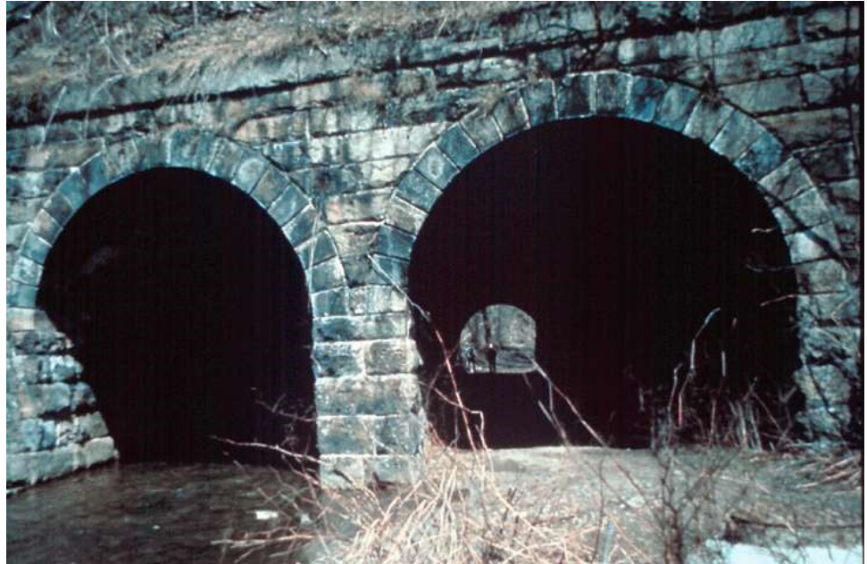
Figure 14.1.15 Stone Masonry Arch Culvert
